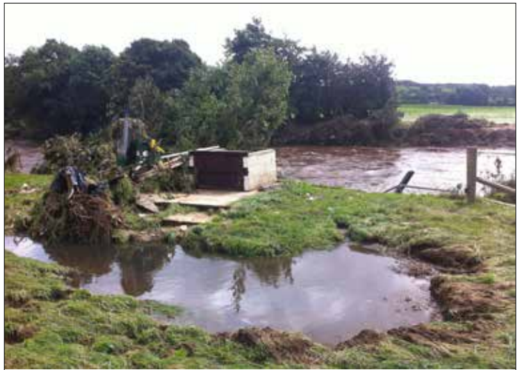
Fig. 1 Demolished gauging hut on the River Owenkillew at Crosh (Northern Ireland) following the extreme flood on August 22nd. (Photo: Gary Galbraith, Rivers Agency).
