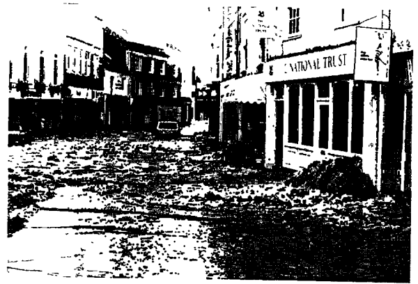
Plate 2. Surcharging of manholes in River Street, Truro during the October 1988 flood.
