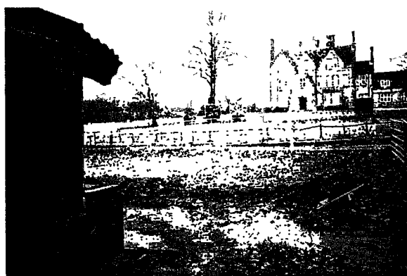
Plate 1 Chilgrove House borehole overflowing, January 1994 Photo: Phillip Turton
