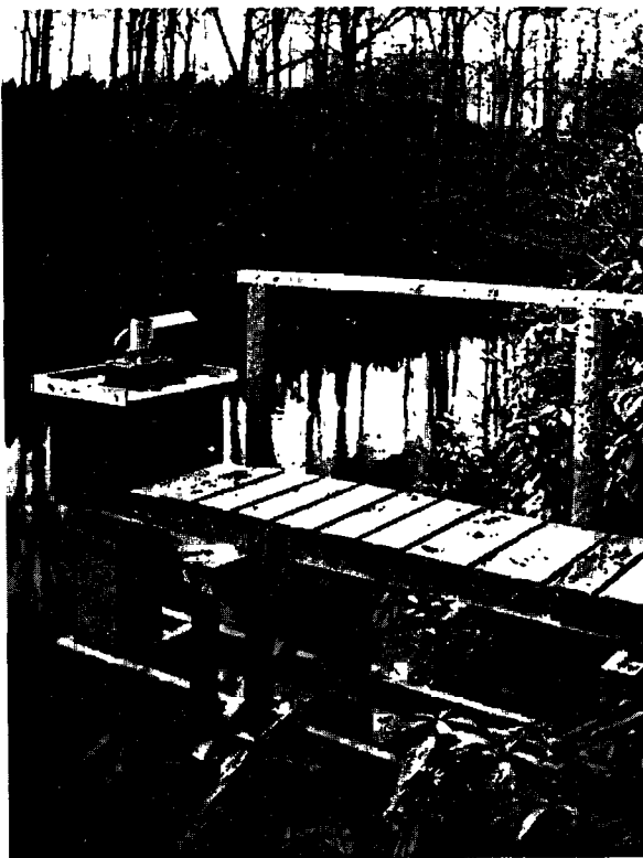
Plate 1. Water level recorder installed at Invergarry Lodge, Invergarry - 1913.
