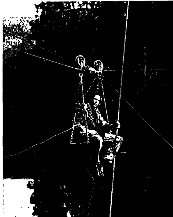
Plate 2. Current metering from a bosun's chair on the River Garry - 1913.
