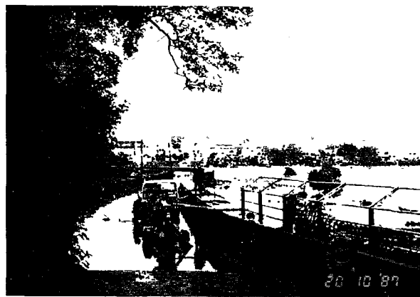
Plate 3. Pumping floodwaters back to the River Tywi over the flood retention wall.
