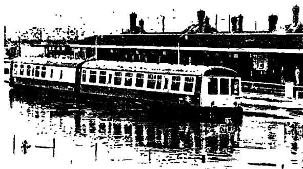
Plate 2. Inundation of Carmarthen Station - 19/10/87.
